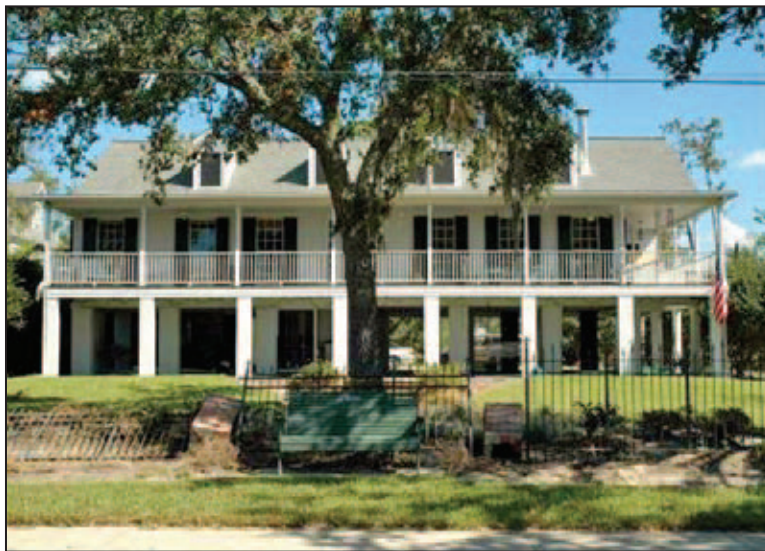
Figure 6-29. Elevation on timber piles
