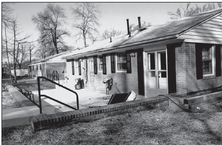
Figure 6-55. Brick-faced residential floodwall and access stairs
