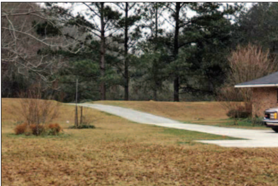
Figure 6-57. Driveway access over a residential levee
