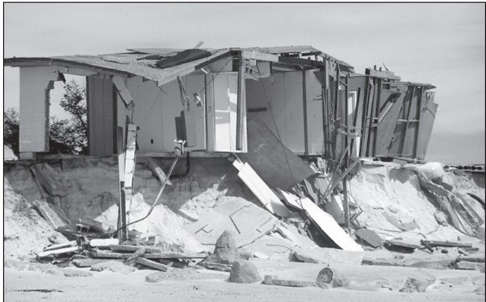
Figure 3-8. Large, fast-moving waves combined with erosion and scour to destroy this Gulf of Mexico home during Hurricane Opal
