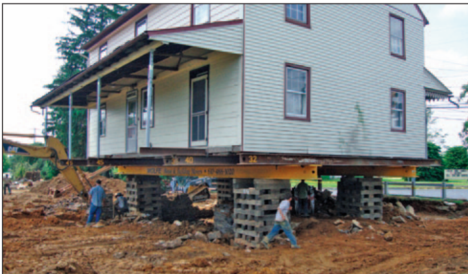
Figure 5R-8. Structure is separated from its foundation (photo courtesy of Wolfe House Movers)
