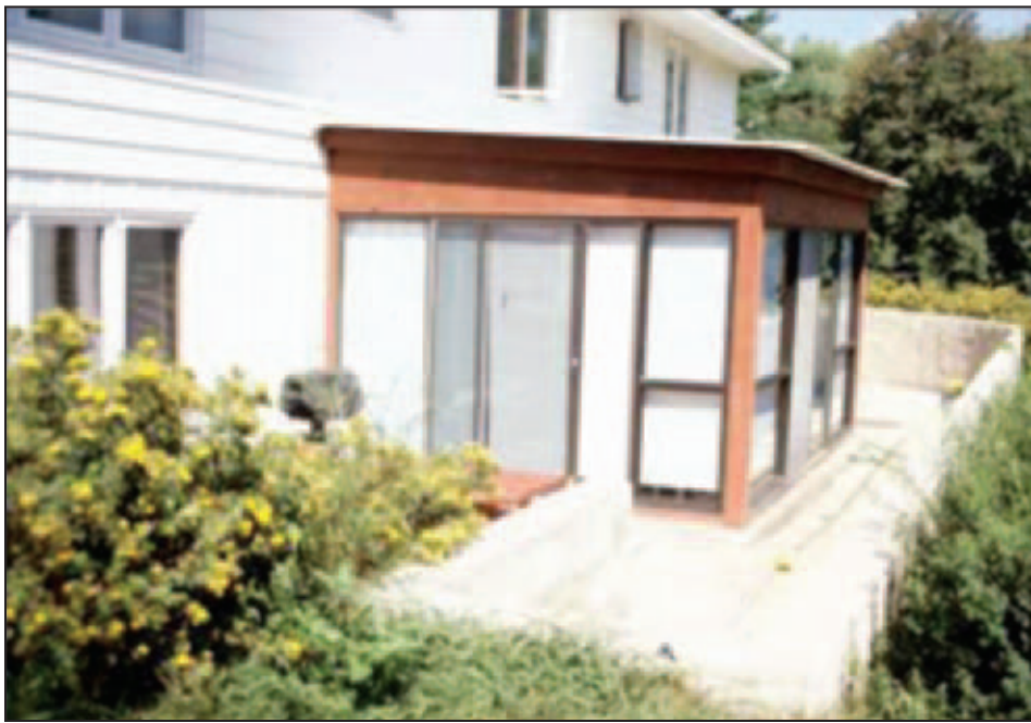
Figure 5F-2. Typical residential floodwall
