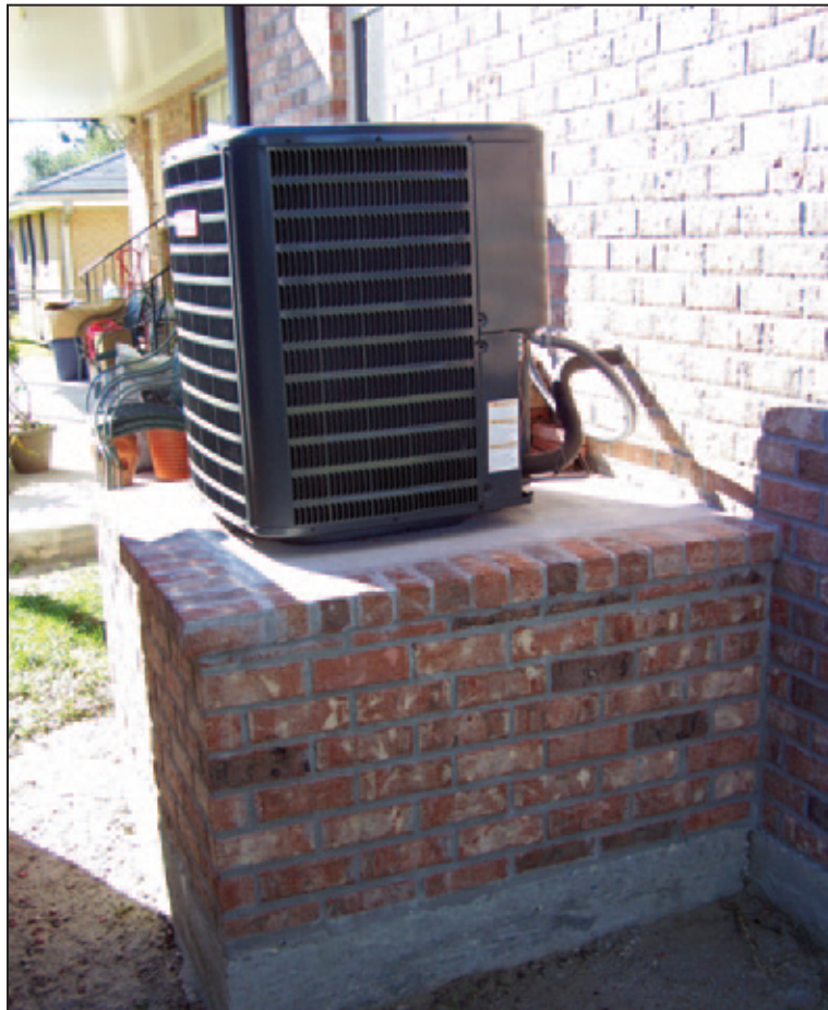
Figure 5W-1. Elevated air conditioning compressor
