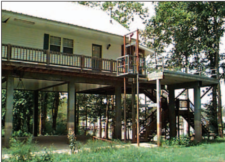
Figure 6-28. House elevated on timber piles
