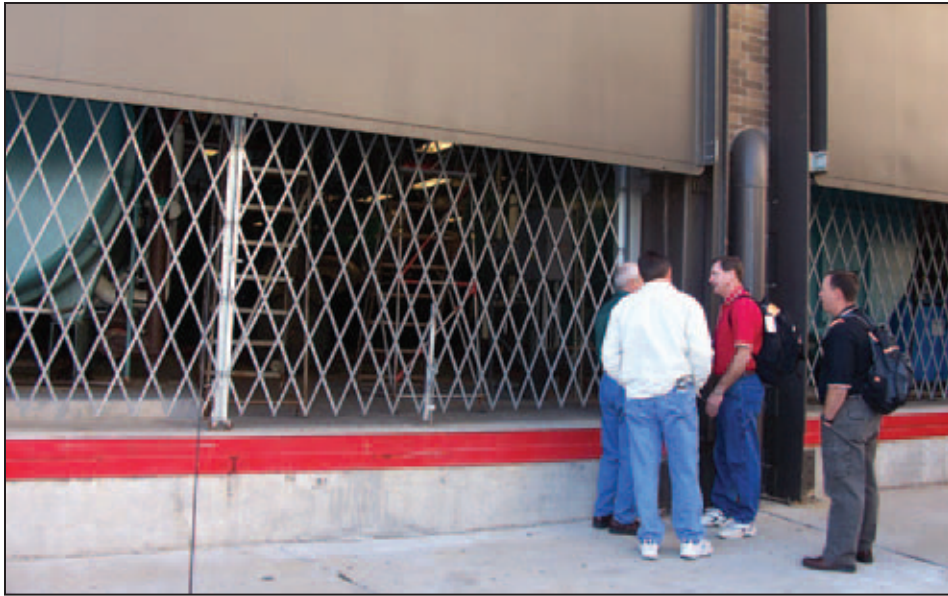
Figure 5D-39. Flood shields that can be raised and lowered to protect a hospital mechanical room from floodwaters
