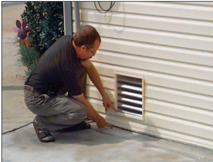
Figure 6-43. Example of flood vents
