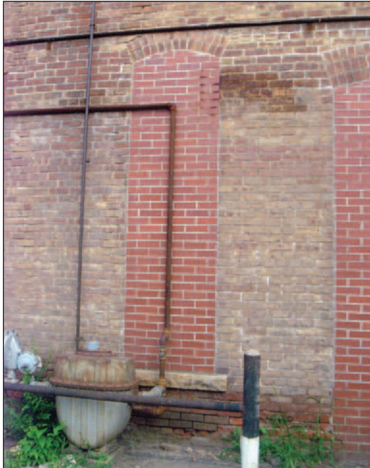
Figure 5D-37. Permanent closure of an opening to prevent floodwaters from entering the building
