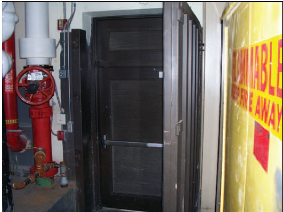
Figure 5D-38. A watertight door used to protect mechanical rooms for a hospital subject to floodwaters
