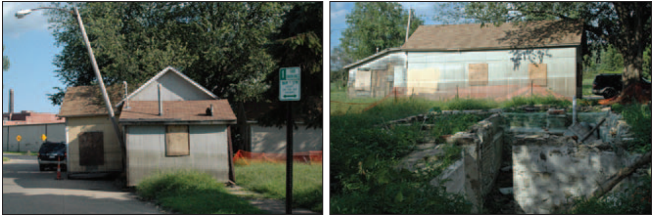
Figures 5D-11 and 5D-12. This house located in the SFHA was displaced from its foundation into the roadway adjacent to it. The photo on the right shows the house's original location.
