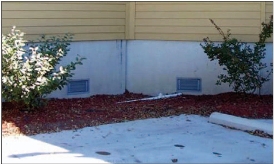
Figure 6-42. Example of flood vents
